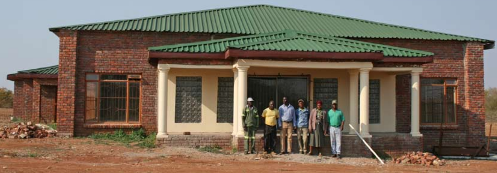
The Community Centre built with Fair Trade premiums nearing completion at Mabunda
